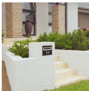
Bagged and painted block work walls
