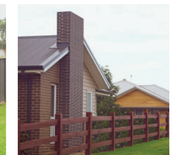
Post and rail fencing, stained dark brown
