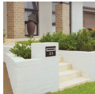
Bagged and painted block work walls
