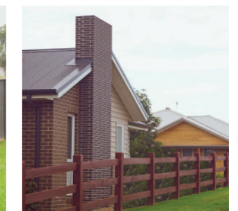
Post and rail fencing, stained dark brown
