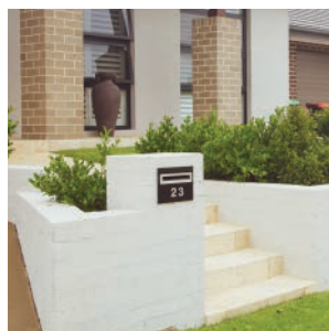
Bagged and painted block work walls
