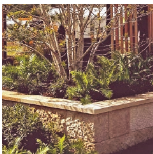
Concrete block clad with natural sandstone tile
