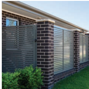
Face-brick with stone capping and metal batten fence in-fill
