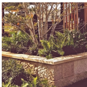
Concrete block clad with natural sandstone tile
