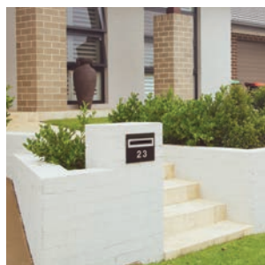
Bagged and painted block work walls
