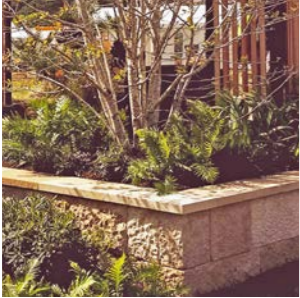
Concrete block clad with natural sandstone tile
