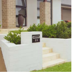
Bagged and painted block work walls
