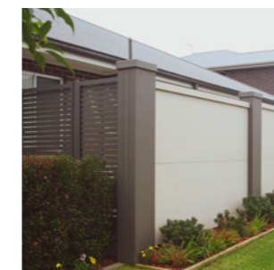
Rendered and painted masonry piers with solid fence in-fill.
