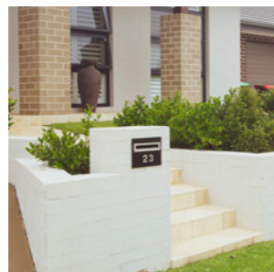
Bagged and painted block work walls
