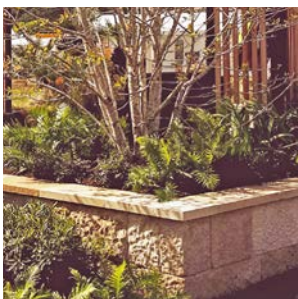
Concrete block clad with natural sandstone tile
