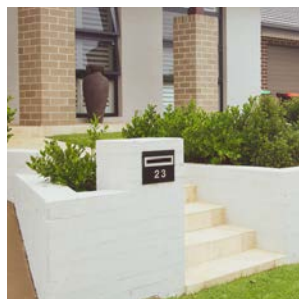
Bagged and painted block work walls
