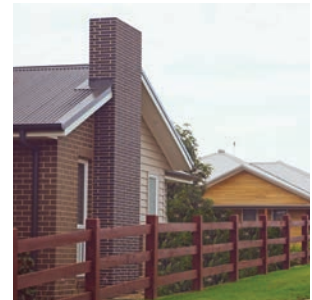
Post and rail fencing, stained dark brown
