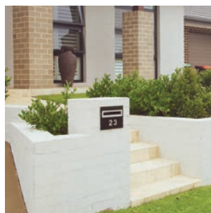
Bagged and painted block work walls
