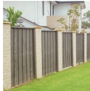
Face-brick with capping, with painted lapped and capped timber in-fill
